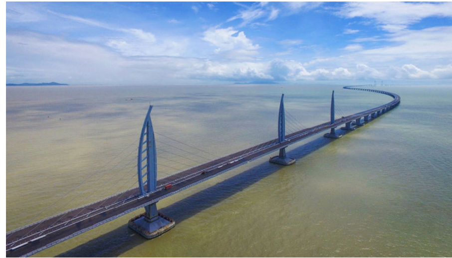
Hong Kong Macao Zhuhai Bridge (China) 55km
