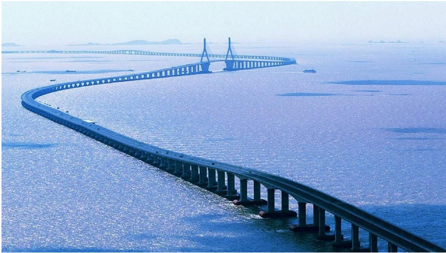
Jiaozhou Bay Bridge (China) 26,7 km
