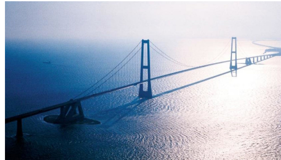
Great Belt Bridge (Denmark) 26,7 km
